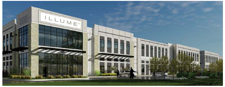
Arbor Lakes 10500 - Maple Grove, MN 277,222-square-foot, build-to-suit headquarters/manufacturing/warehouse facility for ILLUME
