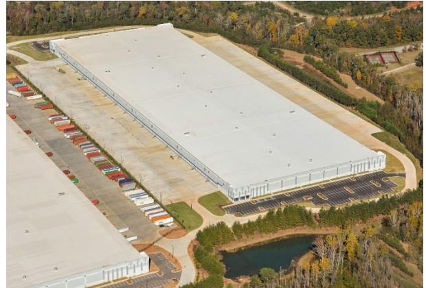
King Mill Distribution Center – Atlanta, Georgia
