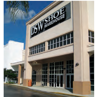
Tower Shops Davie, FL
