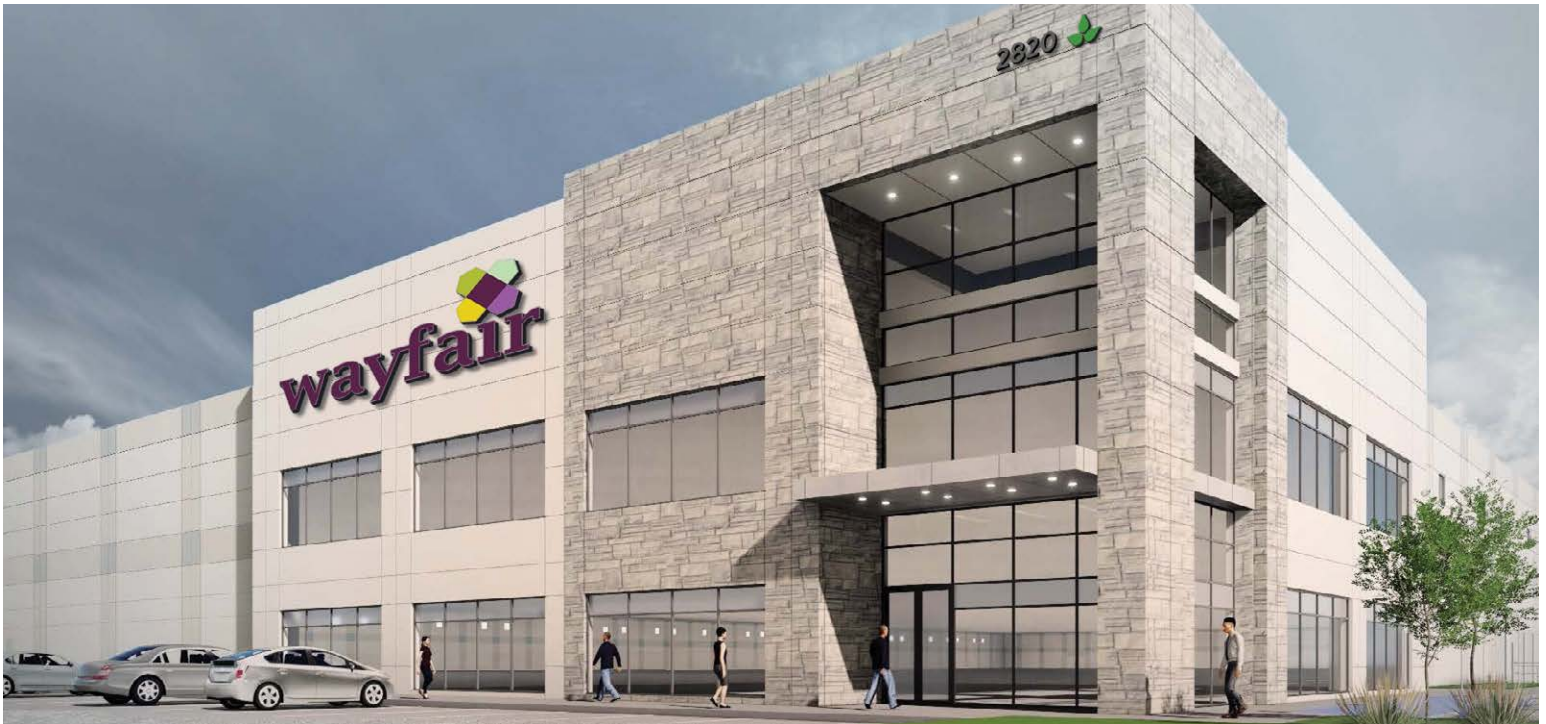
Lancaster 2820, Dallas, TX - 874,566-square-foot, build-to-suit distribution center for e-commerce home goods retailer
