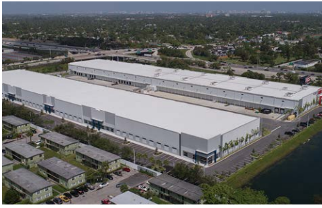
Interstate 95 Center of Commerce – Fort Lauderdale, FL Two industrial buildings totaling 306,465 square feet; 90% leased
