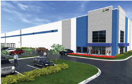
429 Delancy – Newark, NJ 659,000-square-foot speculative warehouse
