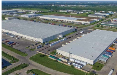
Bayport North Distribution Center – Houston, TX Two industrial buildings totaling 772,500 square feet; 100% leased
