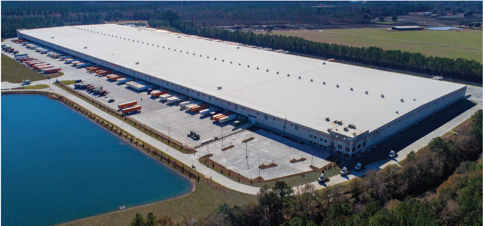
Morgan Business Center 400, Savannah, GA - 1,435,750-square-foot, build-to-suit distribution center for Floor & Decor
