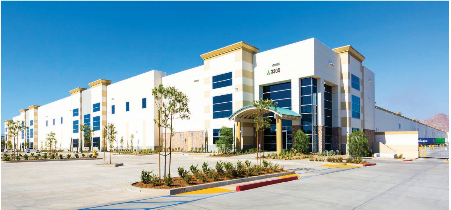
3300 Indian Avenue, Perris, CA - 1,224,874-square-foot, BTS distribution center for home goods e-commerce company; delivered Q2
