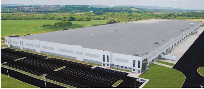
33 Logistics Park – Lehigh Valley, PA 1,015,740-square-foot, speculative warehouse
