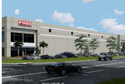
7133 Municipal Drive – Orlando, FL 170,428-square-foot BTS warehouse for PODS Enterprises, LLC
