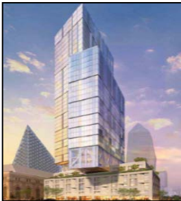
$105MM mezz loan NYC condo construction ~ 13% IRR (3) ; 60% LTV
