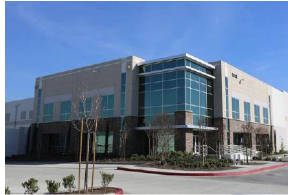
Hofer Ranch Distribution Center Inland Empire West
