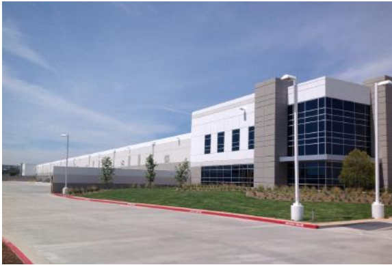
Chino Distribution Center Inland Empire West
