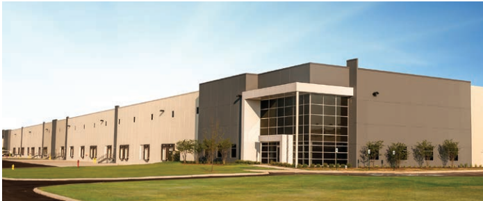
AllPoints at Anson 7A – Whitestown, IN New 257,030-square-foot lease; brings building to 100% occupancy
