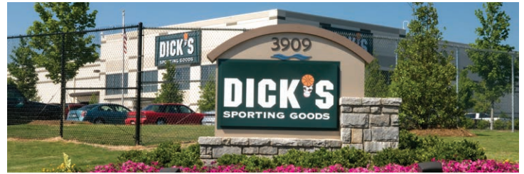
3909 North Commerce Drive – Atlanta, GA 256,600-square-foot expansion of Dick's Sporting Goods built-to-suit distribution center
