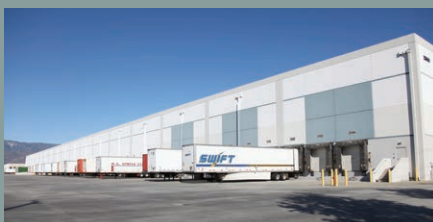
Redlands Commerce Center – Inland Empire, CA 575,457-square foot industrial building; part of a 4.86 million-square foot portfolio acquisition
