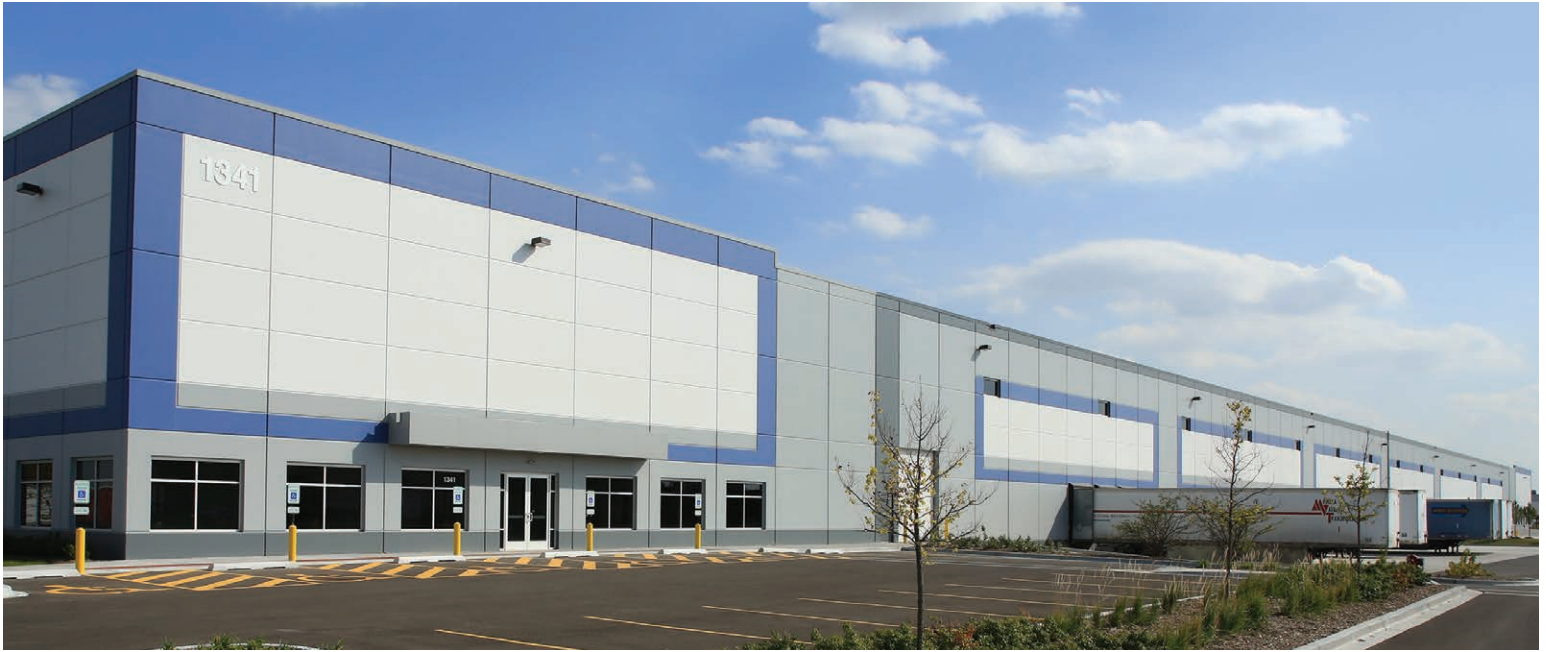
1341-1343 Enterprise Drive, Chicago, IL — 324,115-square-foot speculatively developed warehouse; 78% leased upon completion.
