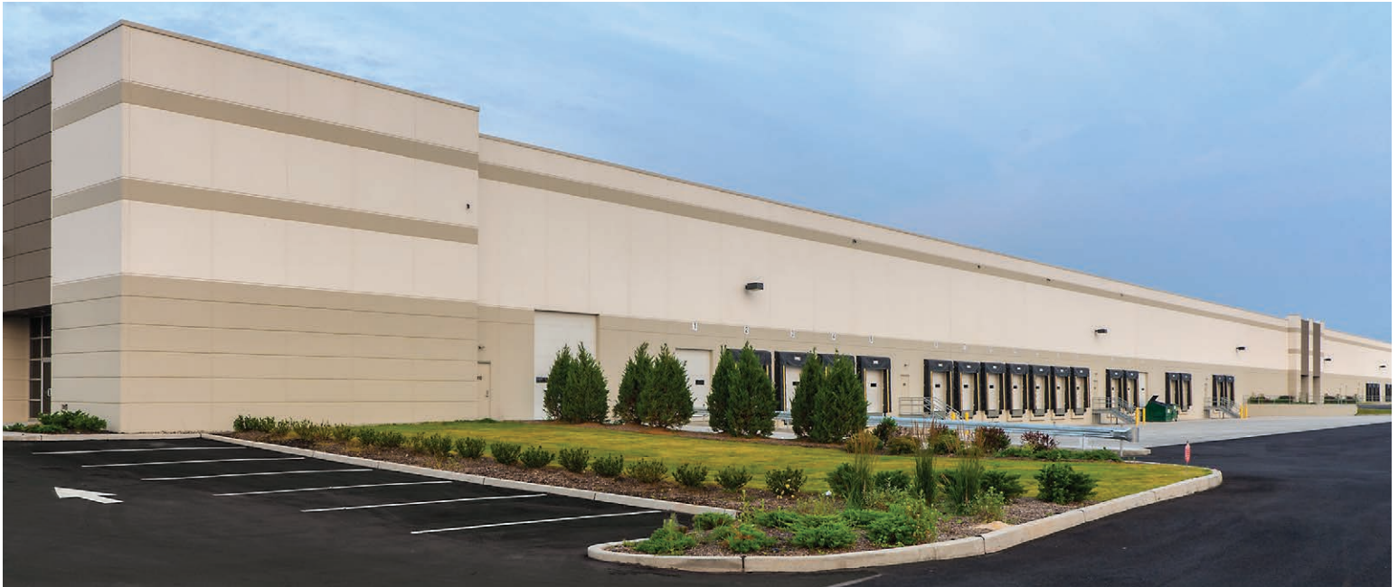
Legacy Commerce Center, Linden, NJ — 301 Pleasant Street, 144,000-square-foot, speculatively developed warehouse 100 percent leased upon completion
