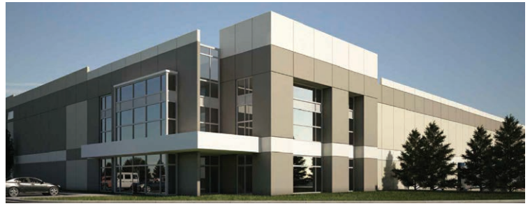
Intermodal North 3 – Rickenbacker Global Logistics Park, Columbus, OH 482,220-square-foot speculative industrial building; 53% preleased to INNO-PAK
