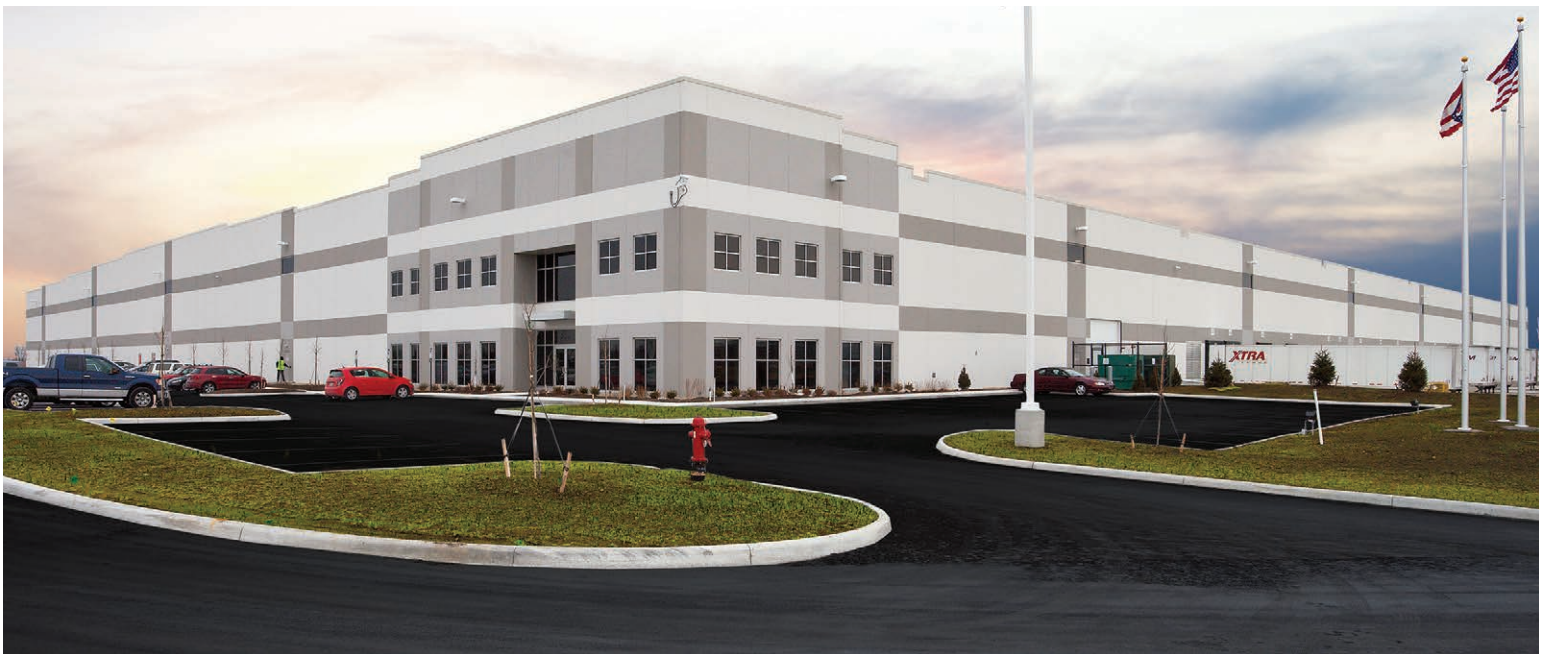
Rickenbacker Global Logistics Park, Columbus, OH — 304,560-square-foot, build-to-suit warehouse for American Showa, Inc.
