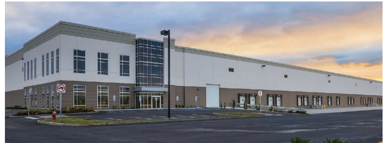
Legacy Commerce Center – Linden, NJ 67% occupancy in two speculatively developed industrial buildings in less than six months
