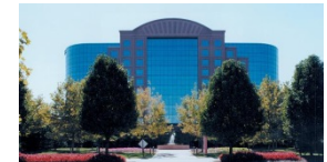
Riverport Tower St. Louis, Missouri
