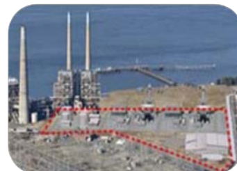
Willow Pass Generating Station
