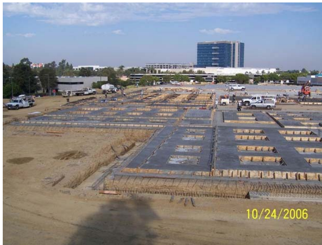
Cardinal Health Campus, Sorrento Mesa, San Diego 318,000 s.f. currently under construction
