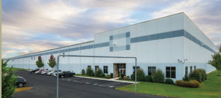
500 Independence Avenue – Mechanicsburg, PA 342,500-square foot, 100% leased industrial building
