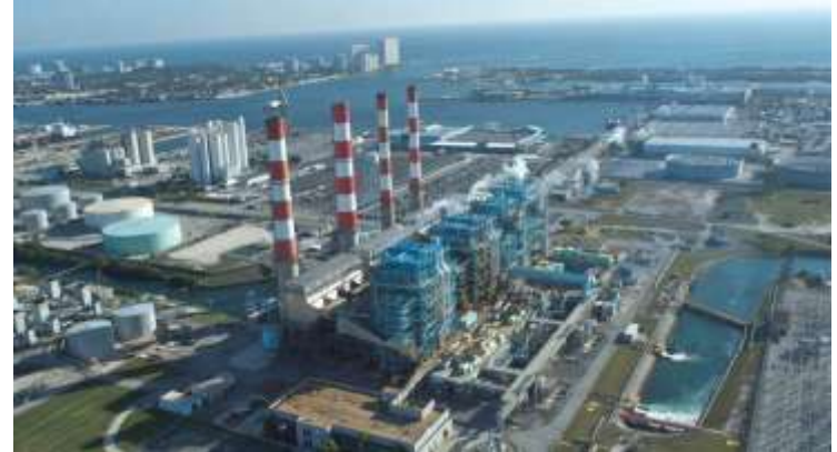
Current Port Everglades Plant
