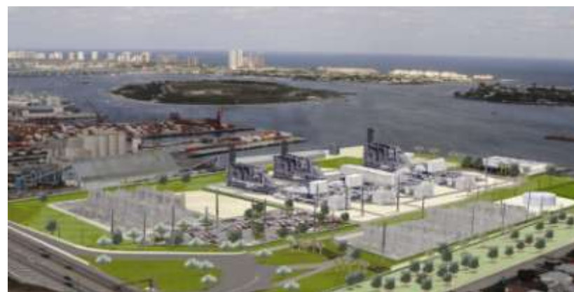
Modernized Riviera Beach Energy Center
