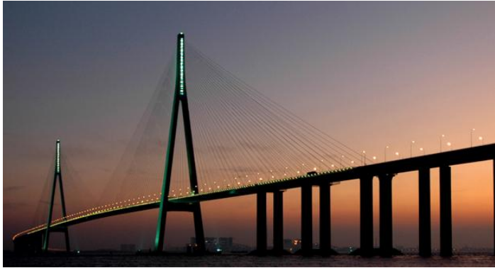
Sutong Bridge Jiangsu, China
